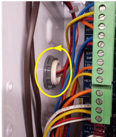
STEP 2: Remove the locknut that holds the base in place.
